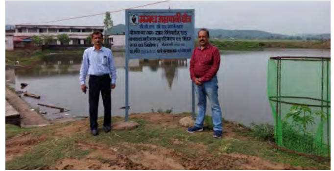
Construction of Pond, Teliyadh, M&A Area
