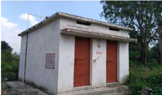
Toilet Constructed under CSR
