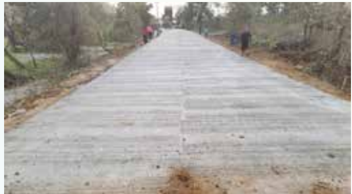
(a) Construction of Road from Dibulganj to Belwadih in Kuldombri
