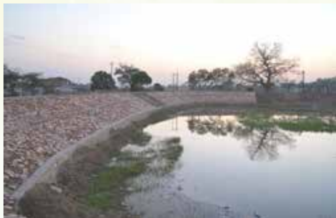
Image 3: Installation of Hand pumps and development of Pond at Gharauli
