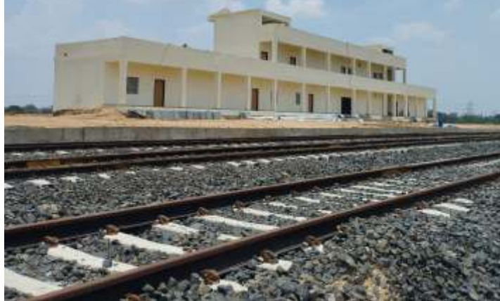
Bhadi Station Building
