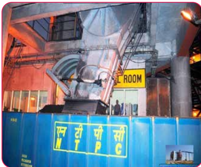
Rake loading in Silo at Dipka Area
