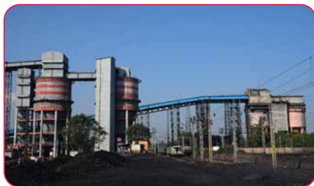
Rapid Loading System-SILO at Gevra Area
