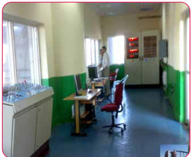
Rake loading Control Room (Silo) at Dipka Area
