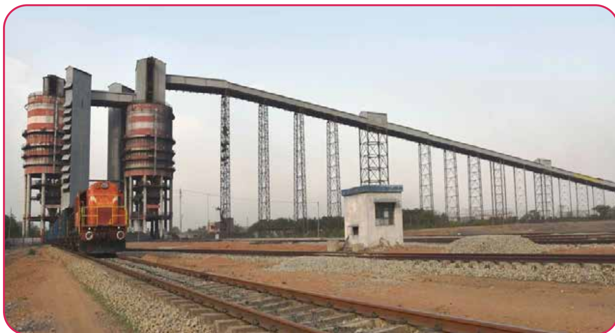
Rapid Loading System (SILO) at Dipka Area
