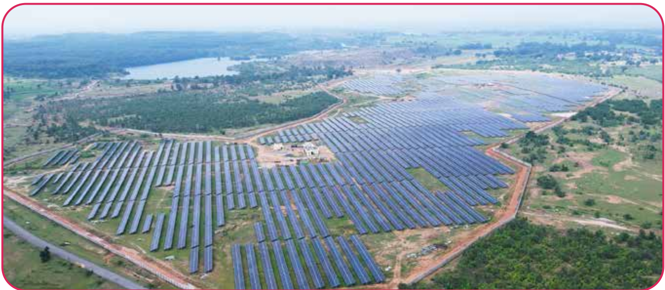
20 MW Solar Plant of Bhatgaon Area
