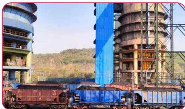
Wagon loading through SILO at Kusmunda Area
