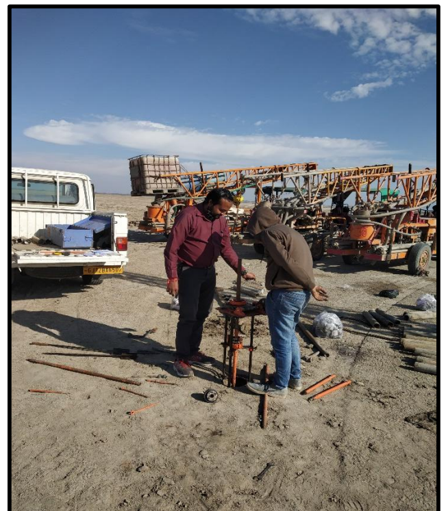
FIELD VANE SHEAR TEST
