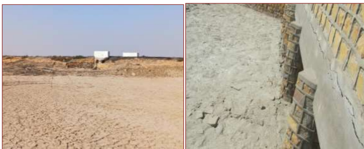
Figure 23: Inter-connected drains between GIPCL project site
