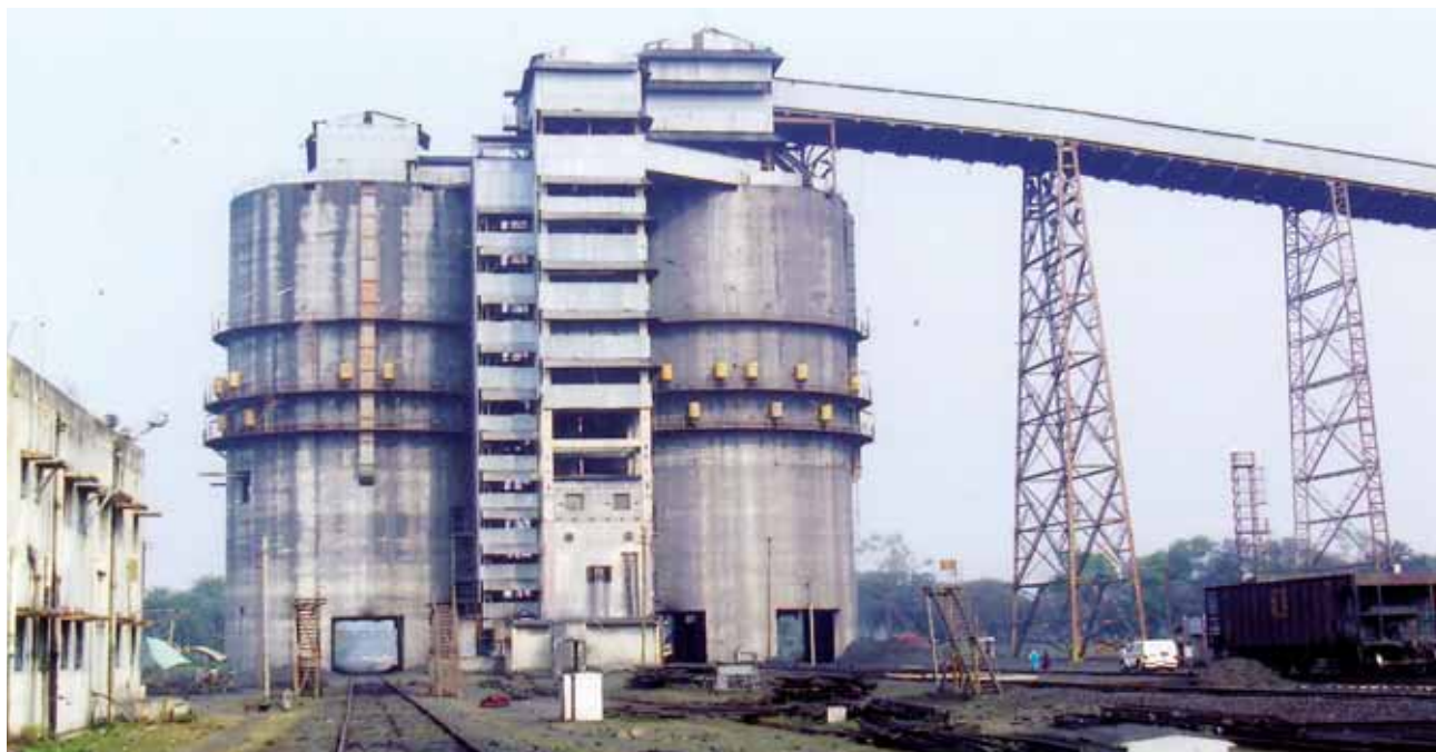
SILO – a computerised system for coal loading directly in Railway Wagons at Coal Handling Plant
