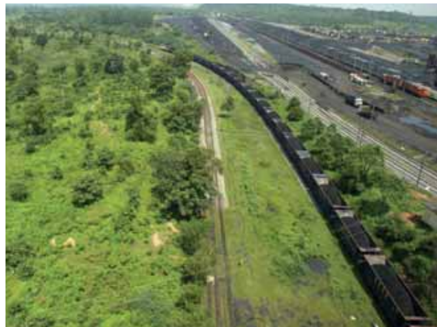
Railway Wagons loaded with coal, coming out from Coal Handling Plant and proceeds towards a Thermal Power Station
